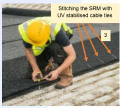
Leave your stitches loose, as over tightening the cable ties will cause buckling of the SRM. The smooth side of the SRM should face uppermost so as to shatter the falling raindrops on impact then allowing the rain water to trickle through the matrix and drip silently on to the roof surface.
