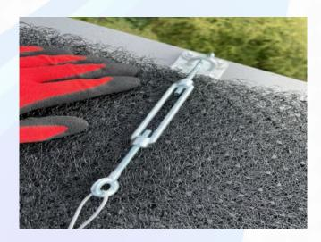
Below is a series of images (not to scale), of the various items utilised when installing Silent Roof Material, restraining wires, turnbuckles, anchors etc. These items are readily available from fencing material suppliers and the like.
