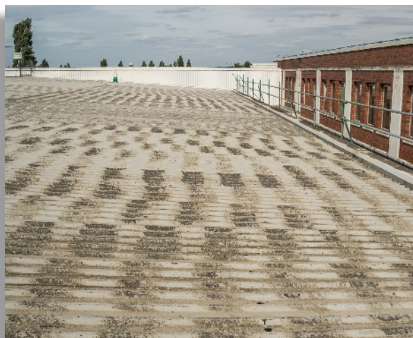
Typical PMR roof structures
